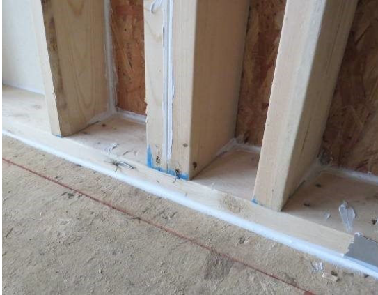
Airsealing wall cavities with Caulking
