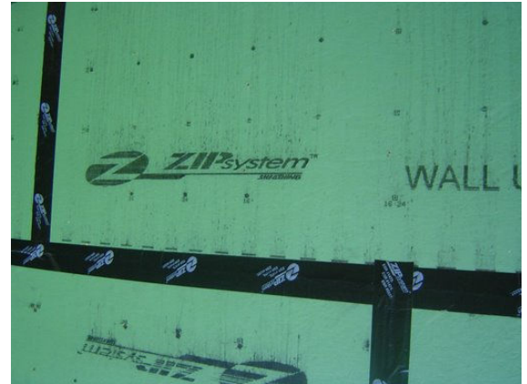
ZIPsystem—Sheathing has waterproof coating, seams are sealed with permanent adhesive tape
